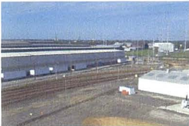
Early construction began in Fall 2013.
