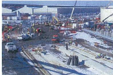
Rail installation and site configuration underway despite snowy conditions in February 2014.
