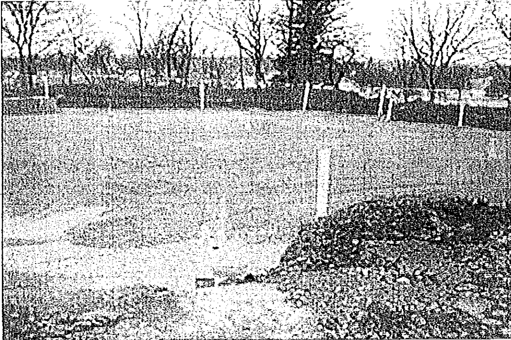
Excavate, level, rock base
