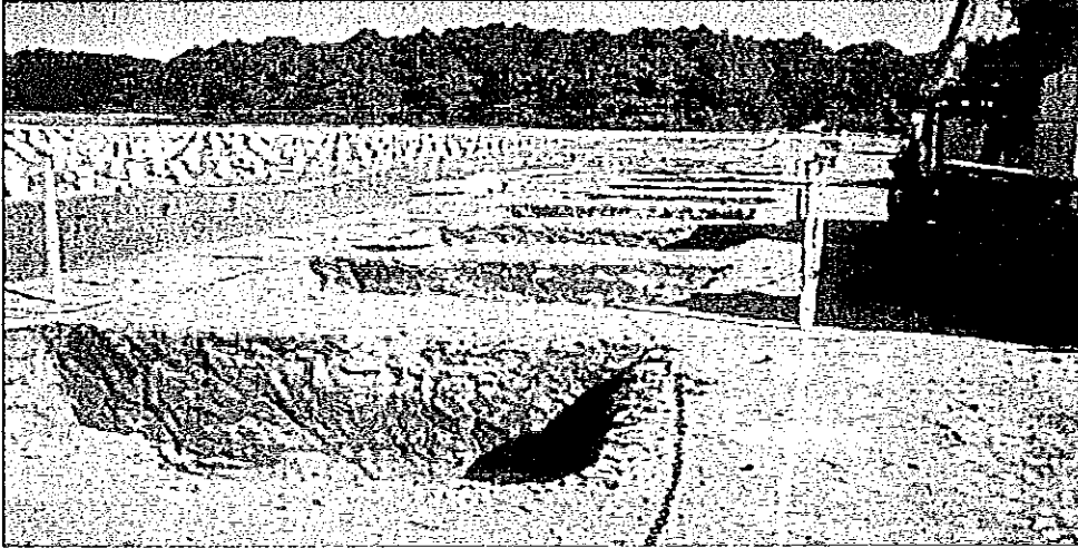
Excavate and store excess soil
