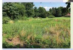
This bioretention basin in West Lampeter Township was constructed two years ago in a portion of an existing detention basin. Water can pond up to 6 inches before spilling into the regular detention basin.
